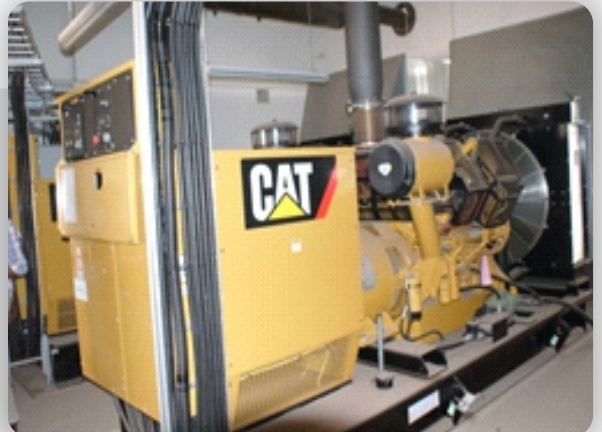
630kVA 400V Gen Set for Brains & Hammers
