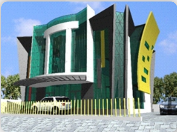
Wuse 2 Office Project, Abuja
