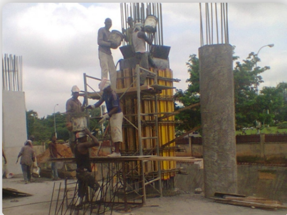
Ongoing Work Progress at Proposed NISA Medical Hospital, Abuja
